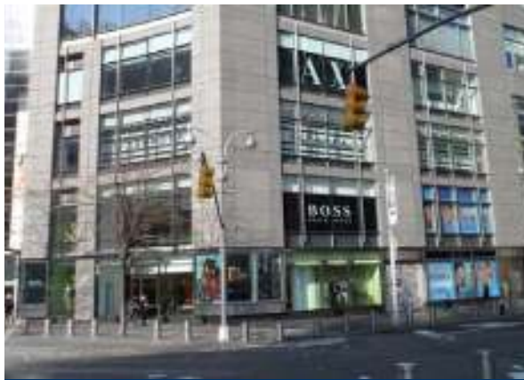
BOSS Store, Columbus Circle // New York, USA (Renovation)
